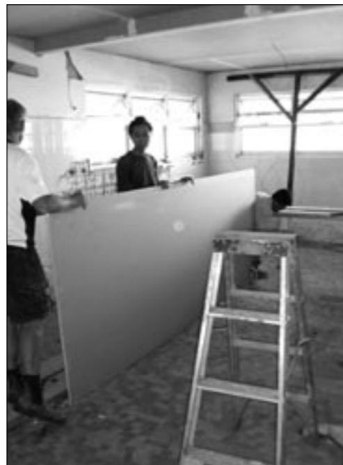
First Year Seminarian, Marlow Domdom from the Philippines assists Mr. Pekolj in hanging gyp-board in the laundry room.
