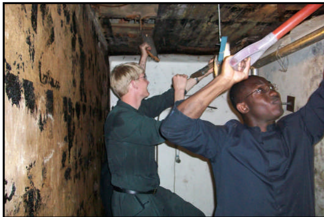
Gutting the walk-in Refrigerators
