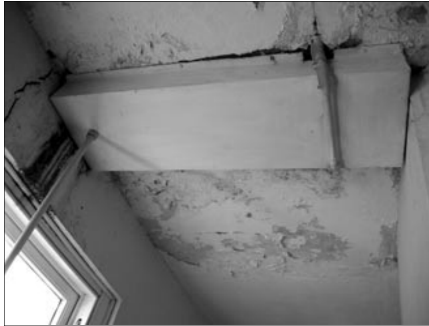
The roof leak and mildew in our Sacristy, needing attention.
